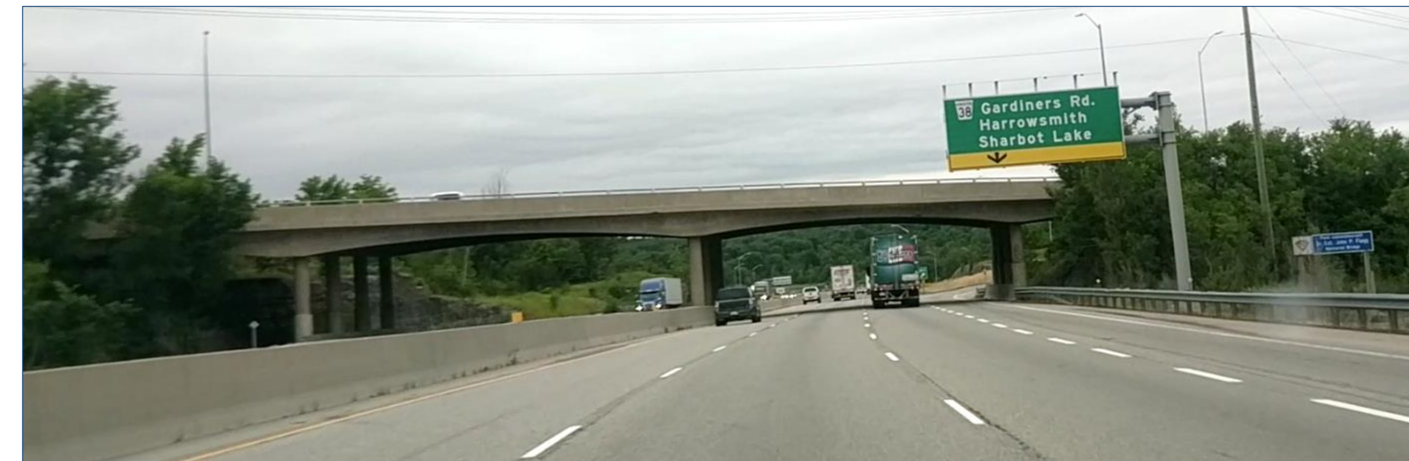
KR 38 Bridge (Westbound)
