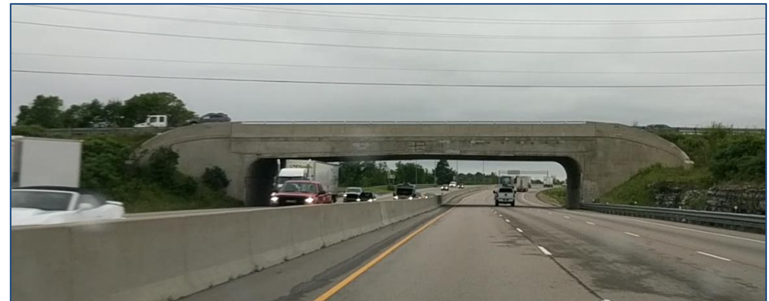
Sydenham Road Bridge (Westbound)
