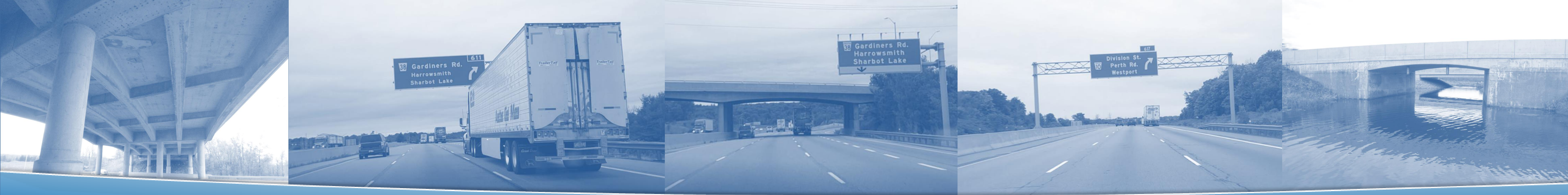
Highway 401 Bridge Improvements at Collins Creek and Interchange/Bridge Improvements at Kingston Road 38 and Sydenham Road
