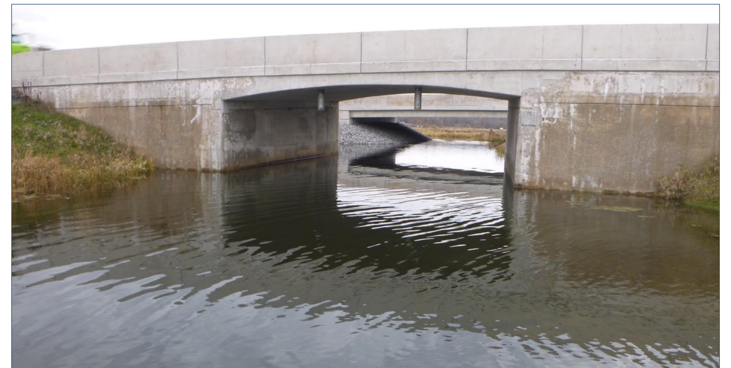
Eastbound Collins Creek Bridge
